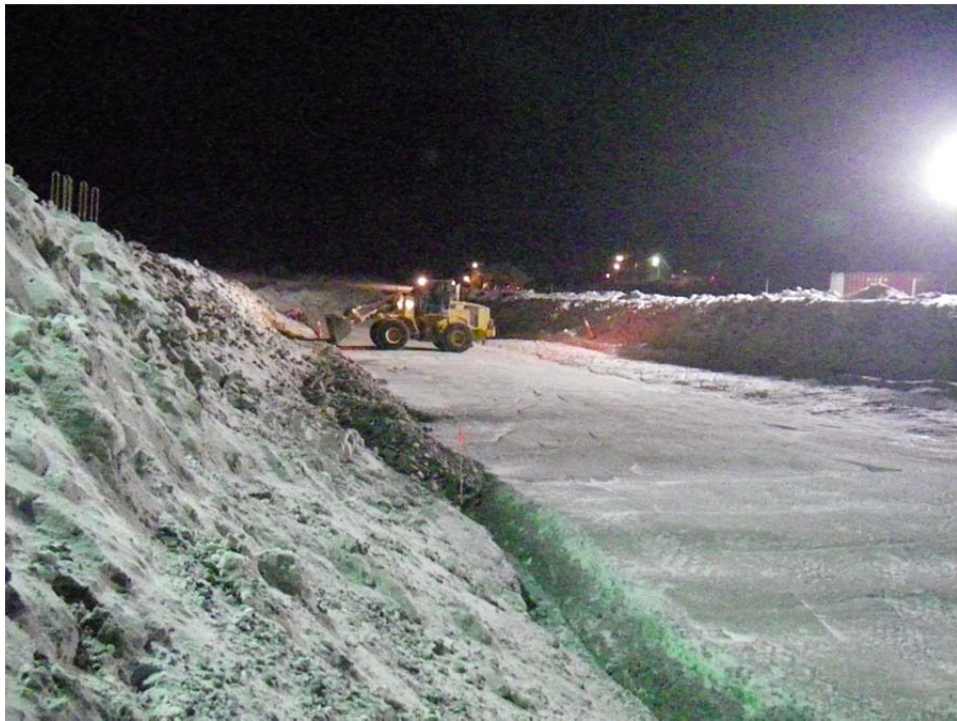
Photo 13: Loader placing transition material along the edge of the key trench. The trough in the forefront of the photo was cleaned and it is planned to be filled with core material.
