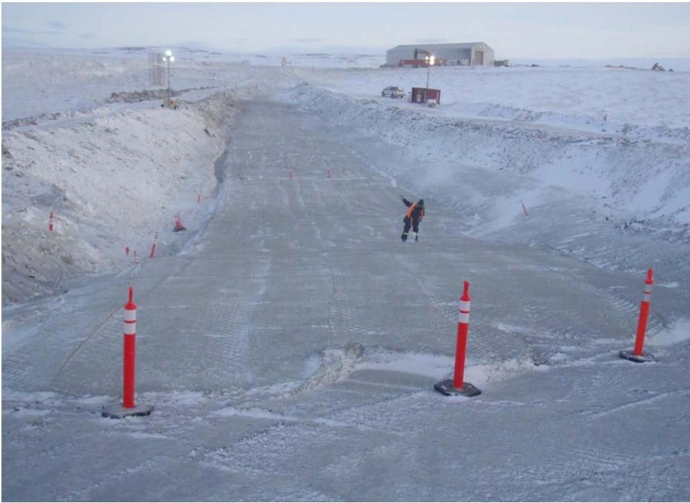
Photo 2: ~ENE view down key trench, EBA taking single bead reading at time of photo.
