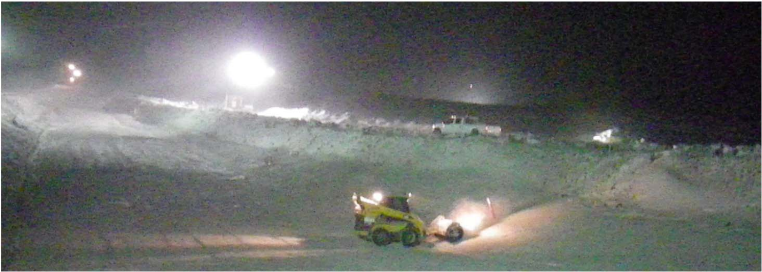
Photo 16: Skid steer with brush sweeping key trench near the end of nightshift.
