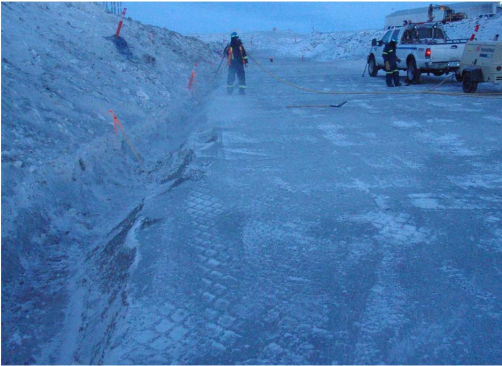
Photo 3: ~ NE view of labourer cleaning slightly underbuilt downstream slope area. See photo 10 for additional details.
