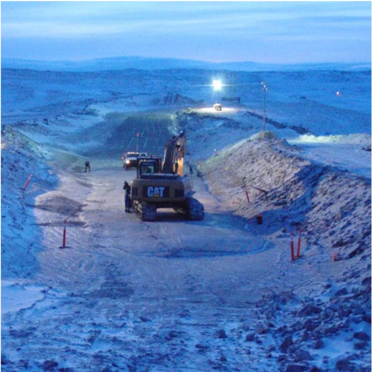
Photo 11: Excavator working on clearing 5/8" clear, and cleaning along the upstream and downstream slopes. ~ WSW view.
