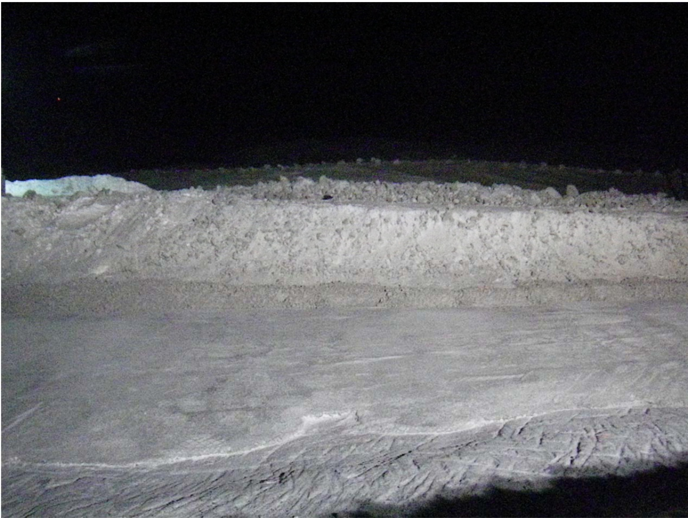
Photo 14: Transition material placed along edge of key trench.
