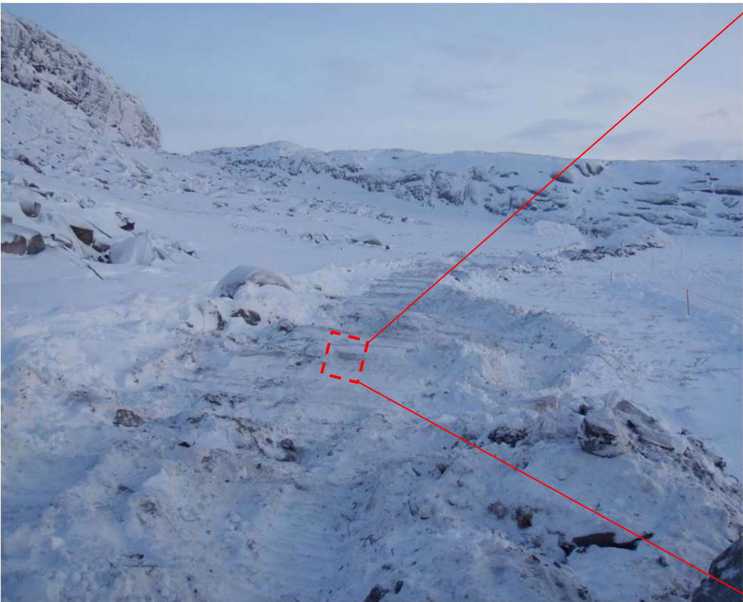
Photo 5: ~~E view down snow clearing completed along DN Diversion Berm footprint. Looking towards E bedrock slope tie-in.
